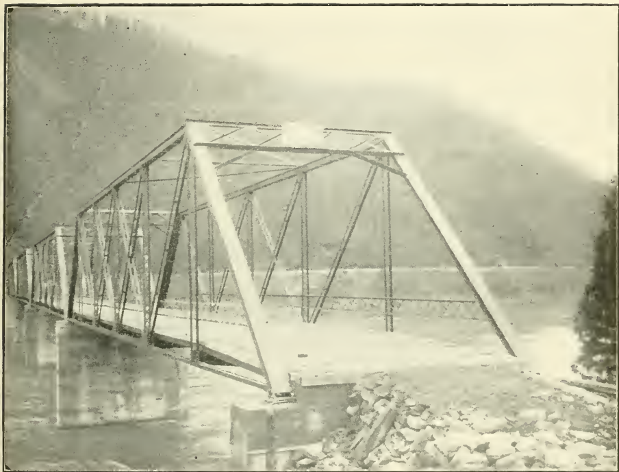
FOSS BRIDGE, Built by Charles Louis Miller, 1907.
